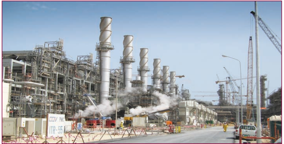
Silent steam blowing to clean pipework
